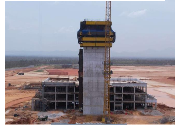
Air Traffic Control Building
