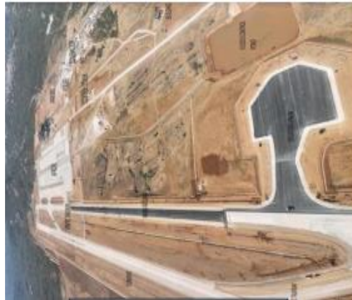
Taxiway Asphalt Paving
